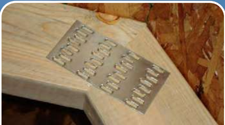
Metal Truss Plates Provides superior strength than wooden gussets.
