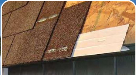
Aluminum Dripedge Added protection against rain, snow, and ice.
