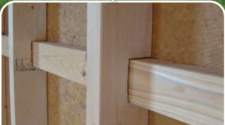
Strongback Nailer A unique Alpine feature, this nailer allows for straighter and stronger walls and siding.
