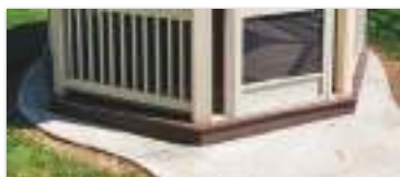
Concrete Pad or Deck
