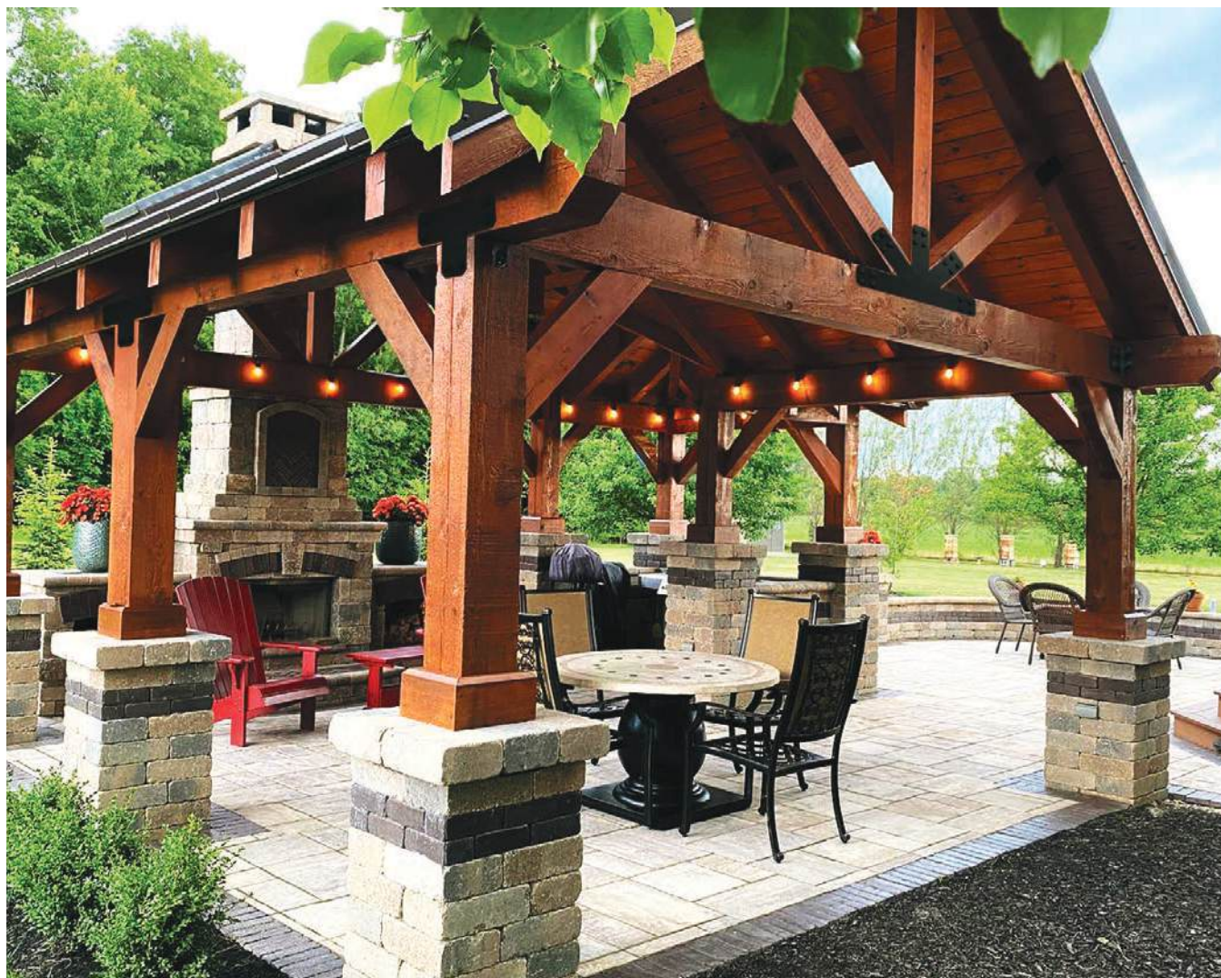
Above: Custom Alpine Pavilion in cedar, cedartone stain, 8" square posts with stone pillars, standing seam metal roof. | Right: Custom Alpine Pavilion in cedar, cedartone stain, 8" square posts with stone pillars, standing seam metal roof. Pictured without brackets.
