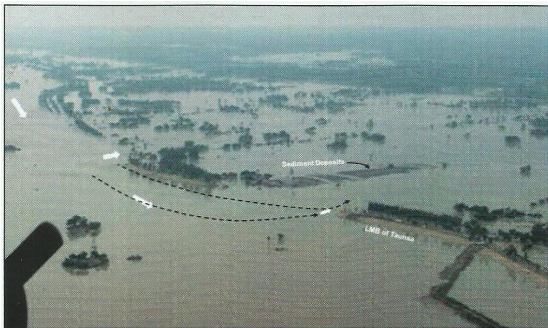
Figure 10: Aerial View of Breach at LMB of Taunsa Barrage
