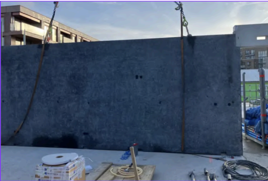
Caption: One of the pre-cast wall elements used in the building. Image used by permission of Voorbij Prefab
