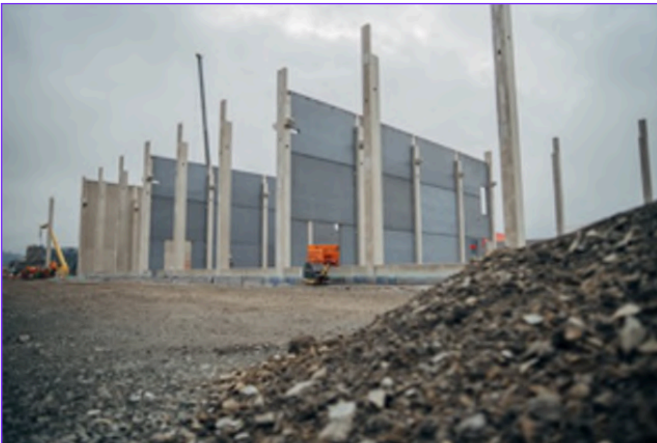
Caption: One of the pre-cast wall elements used in the building. Image used by permission of Voorbij Prefab
