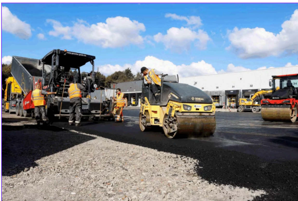
Caption: Carbon neutral asphalt is being laid by Gieseke GmbH. Image used by permission of Gieseke GmbH.
