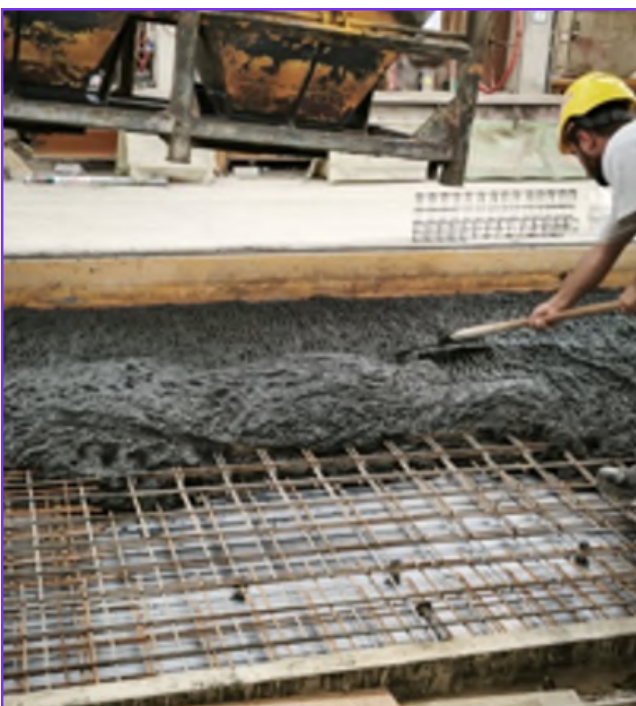
Caption: Concrete-biochar mix is being poured over a rebar form to create a precast wall element. Image used by permission of ecoLocked.
