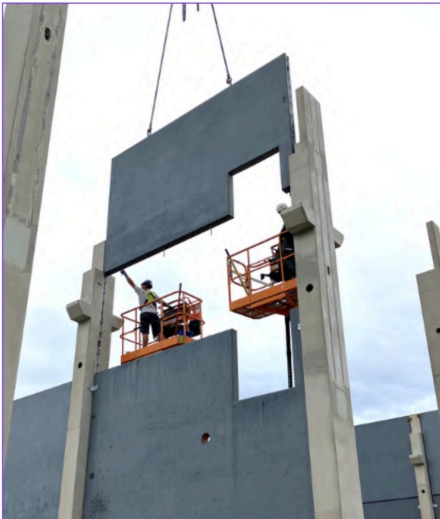
Caption: Precast concrete walls made with biochar admix from ecoLocked are being installed in Kemnath, Germany with construction and engineering company Markgraf. Image used by permission of ecoLocked GmbH.
