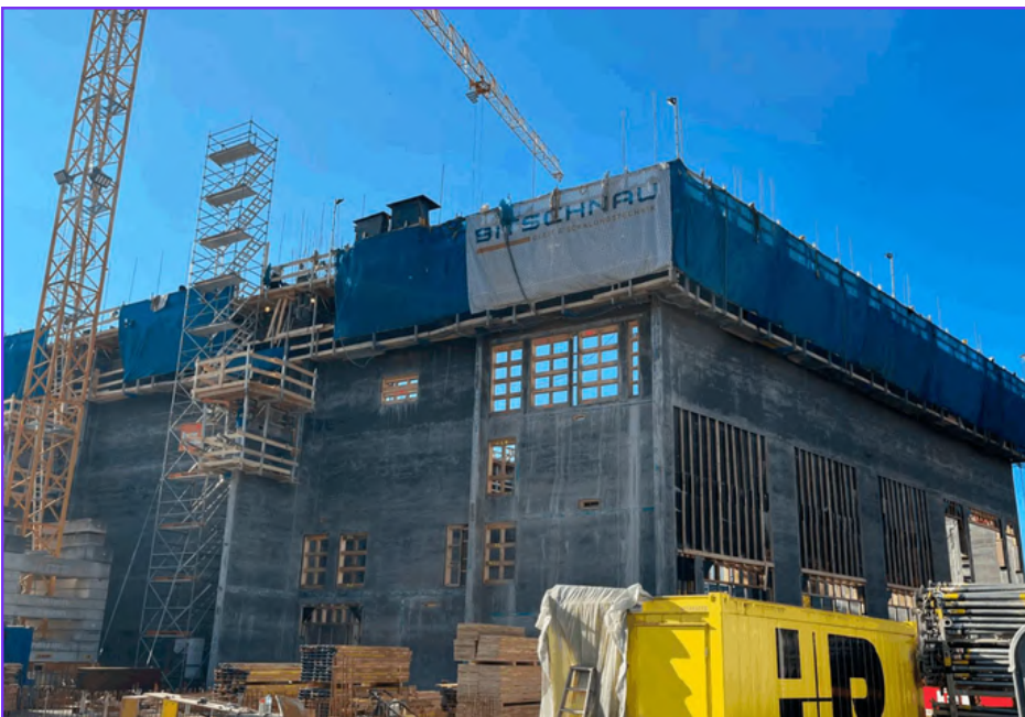
A biochar-concrete mix is being used in a slipform construction, marking the first time in the world this has been accomplished. Image used by permission of CarStorCon® Technologies.
