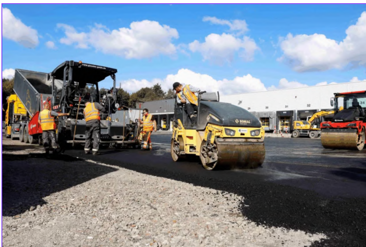
Carbon neutral asphalt is being laid by Gieseke GmbH. Image used by permission of Gieseke GmbH.
