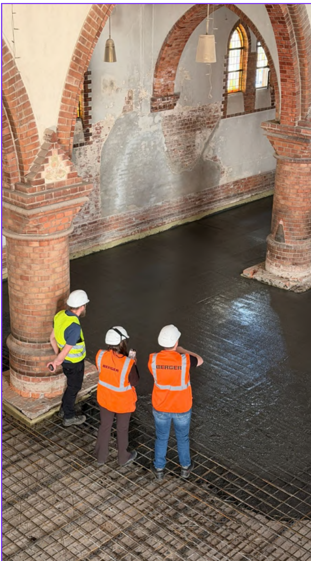
The new, net zero foundation of Johanneskirche as it is being poured. Imaged provided by permission of ecoLocked.
