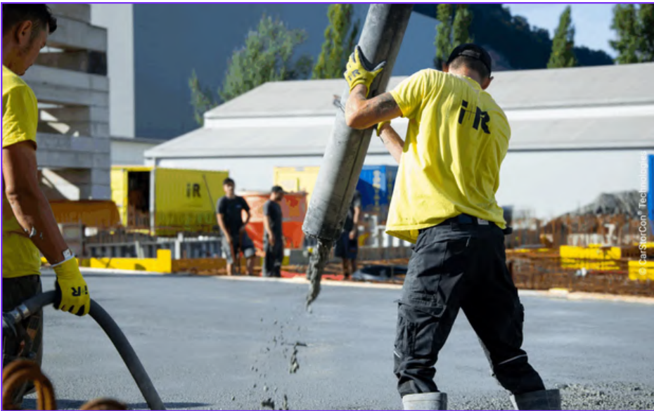
A biochar-concrete mix is being pumped to build the foundation of the new energy plant at Wallenmahd. Image used by permission of CarStorCon® Technologies.
