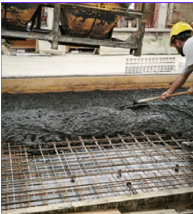
Concrete-biochar mix is being poured over a rebar form to create a precast wall element. Image used by permission of ecoLocked.
