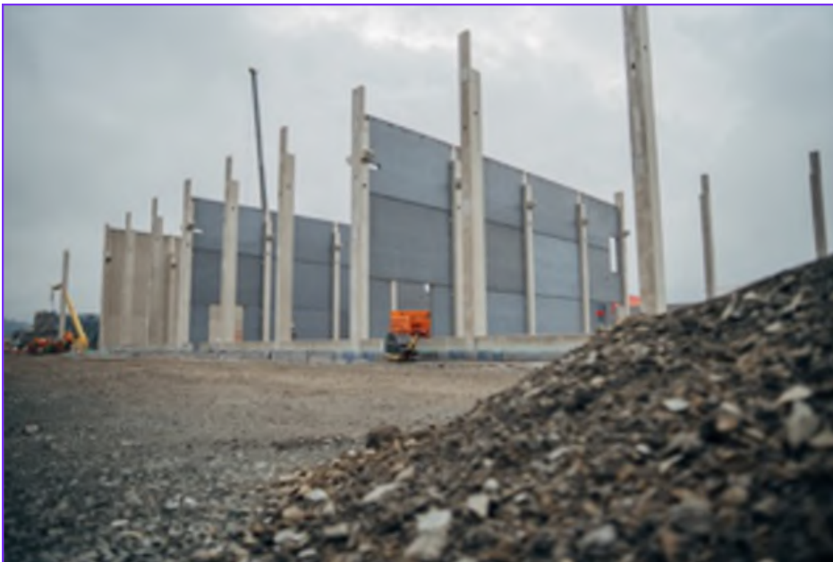
Biochar-concrete precast walls are assembled into a holding structure of a new training and education center in Kanmath, Germany. Image used by permission of ecoLocked.
