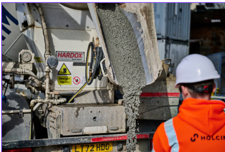
Caption: Ready-mix concrete with biochar is being poured from a concrete truck. Image used with permission of Holcim.
