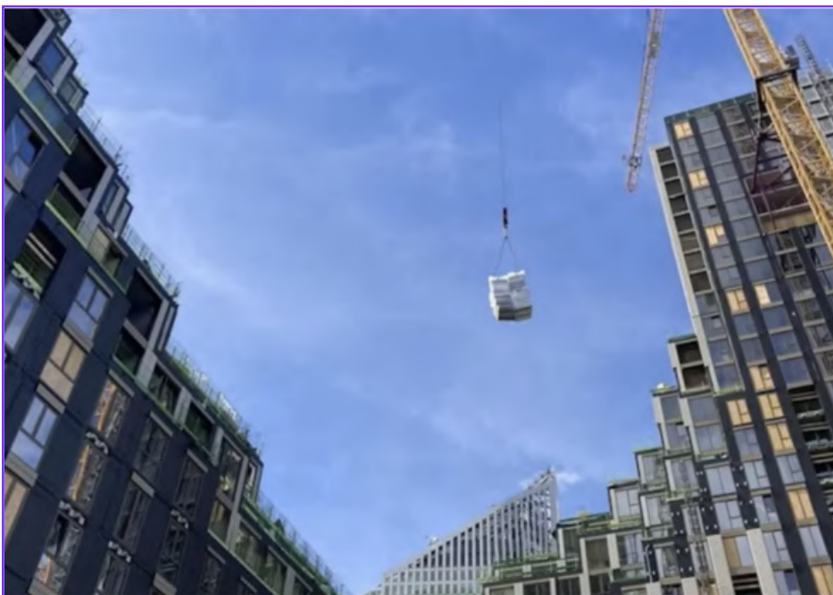
Construction ongoing at the apartment complex in Utrecht, Netherlands. Image used by permission of Voorbij Prefab.
