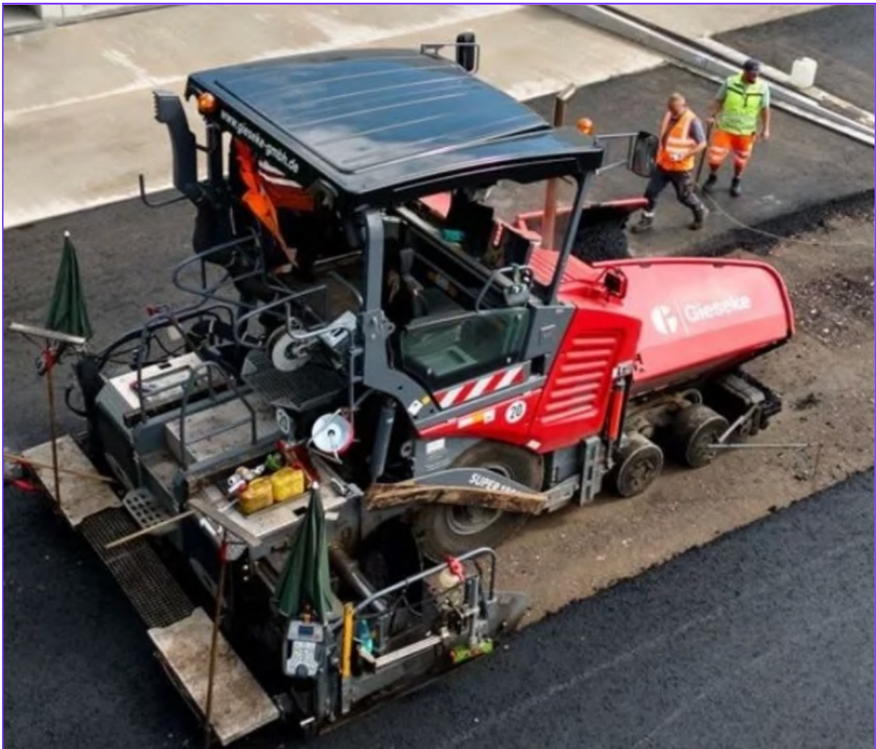
Carbon neutral asphalt is being laid by Gieseke GmbH Image used by permission of Gieseke GmbH.
