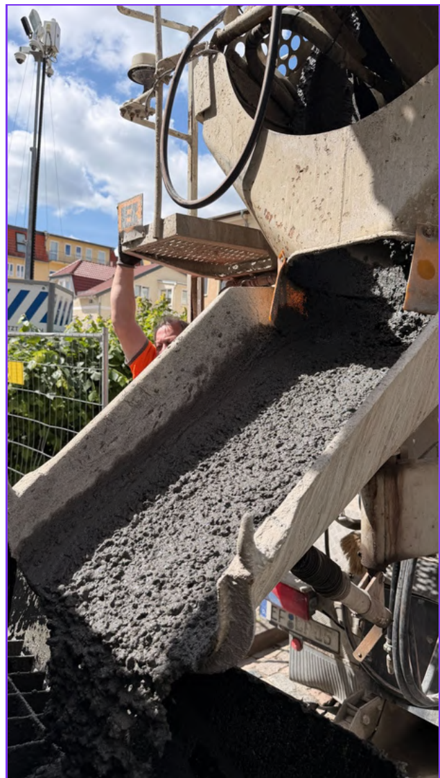
Biochar concrete is being poured at Johanniskirche. Image used by permission of ecoLocked.
