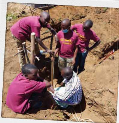
Kids dig the foundation
