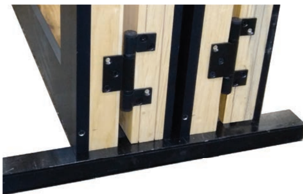
FIG 7: Support Bottom of Panels During Install
