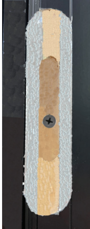
FIG 4 (Minimum of 3 screws per jamb leg recommended)
