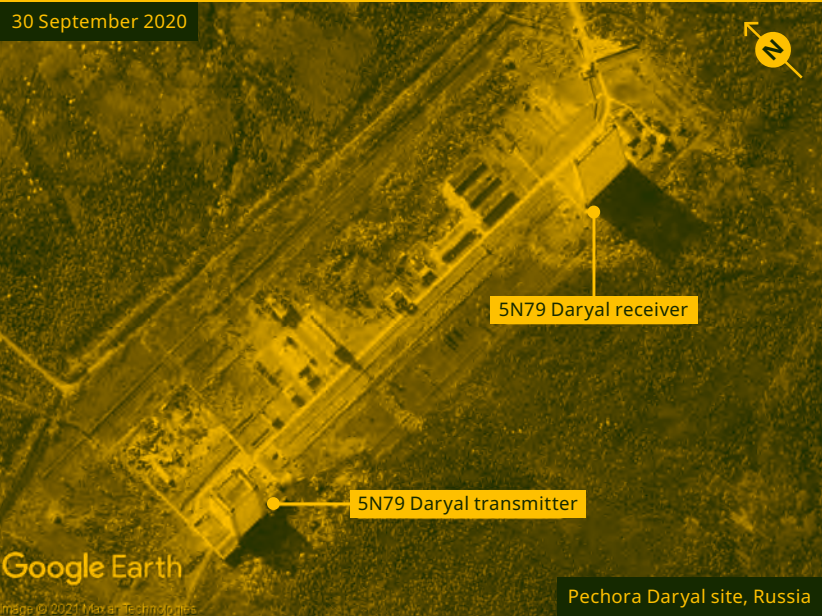
FIGURE 15-42 — DARYAL RADAR AT PECHORA
