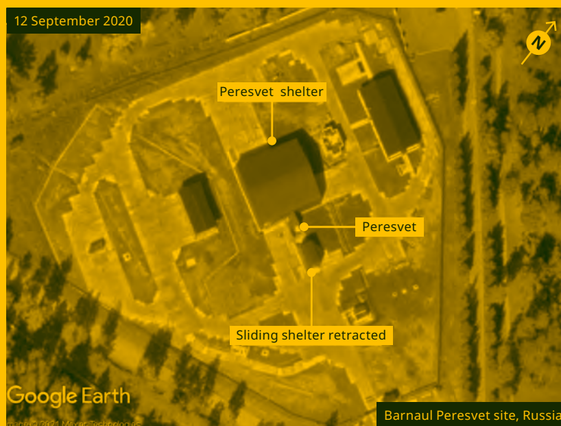
FIGURE 15-25 — PERESVET DEPLOYMENT SITE NEAR BARNNAUL
