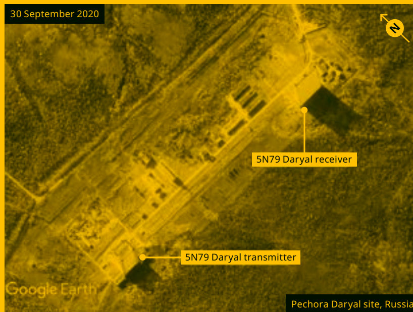
FIGURE 16-43 — DARYAL RADAR AT PECHORA
