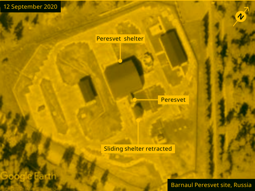
FIGURE 16-26 – PERESVET DEPLOYMENT SITE NEAR BARNNAUL
