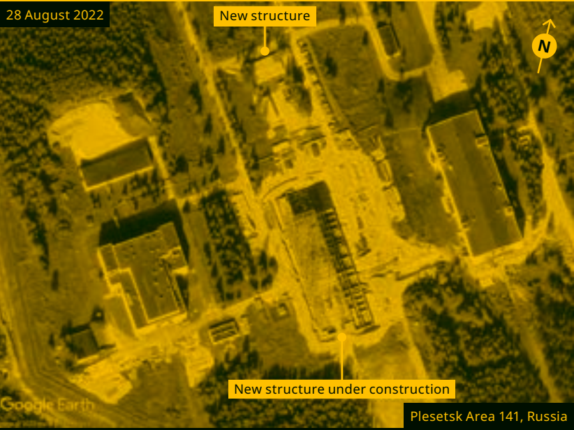
FIGURE 16-8 – PLESETSK AREA 141 BUREVESTNIK FACILITIES
