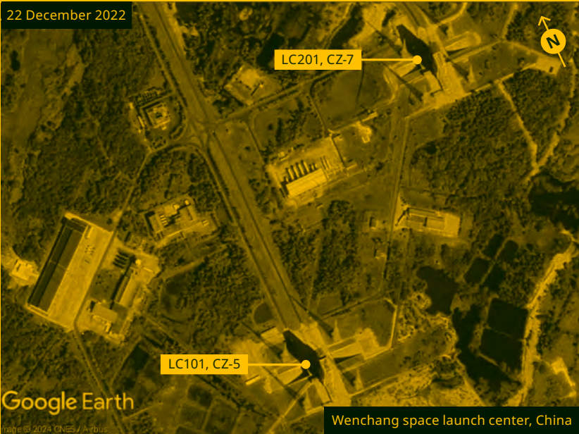
FIGURE 16-15 – WENCHANG SPACE LAUNCH CENTER
