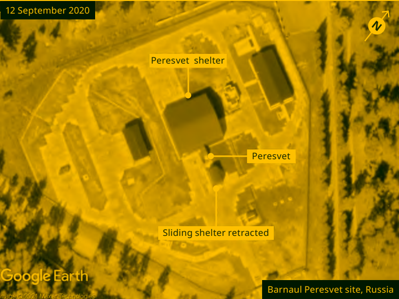
FIGURE 16-26 — PERESVET DEPLOYMENT SITE NEAR BARNNAUL
