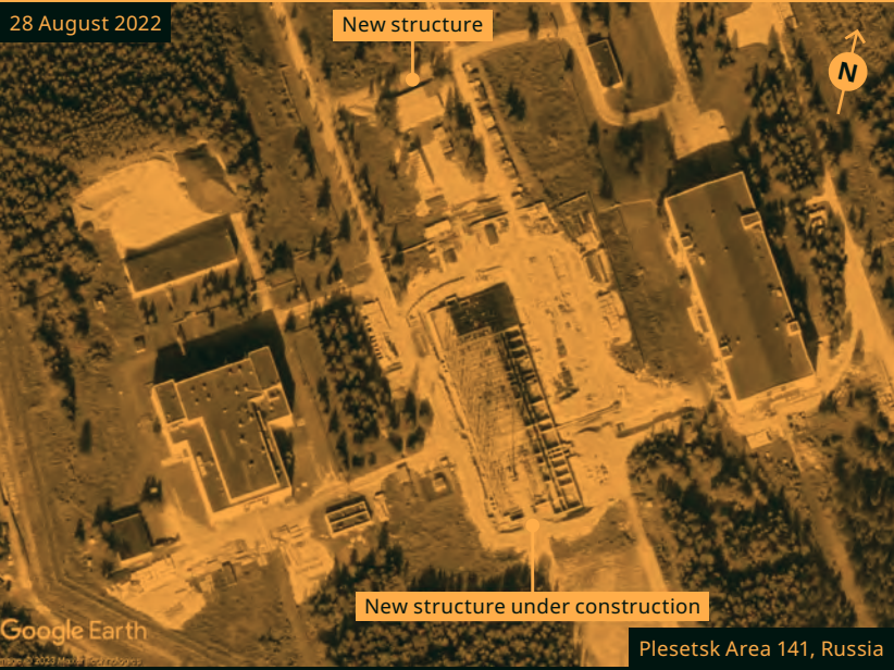
FIGURE 17-8 – PLESETSK AREA 141 BUREVESTNIK FACILITIES
