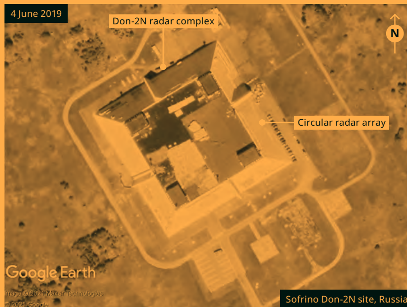
FIGURE 17-45 — DON-2N SITE AT SOFRINO
