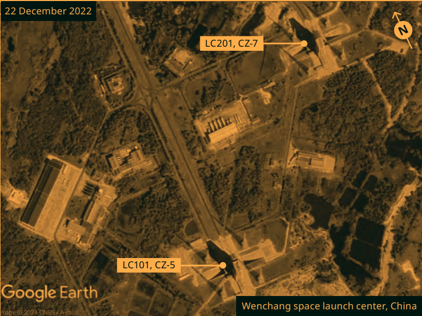
FIGURE 17-15 – WENCHANG SPACE LAUNCH CENTER
