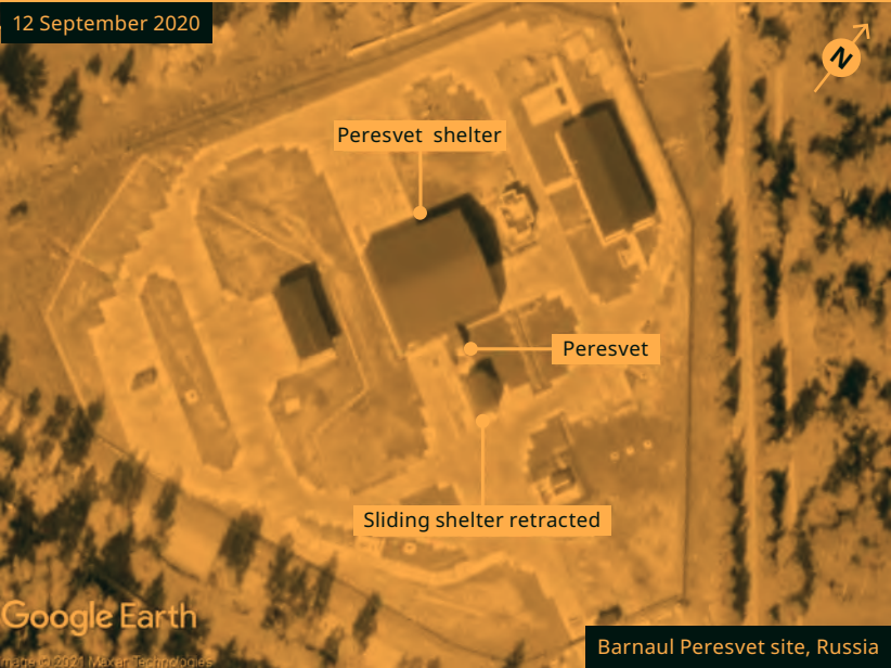
FIGURE 17-26 – PERESVET DEPLOYMENT SITE NEAR BARNNAUL
