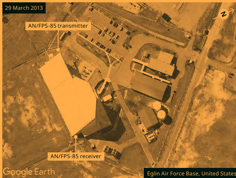
FIGURE 17-33 — EGLIN SPACE SURVEILLANCE RADAR
