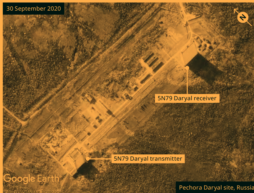
FIGURE 17-43 — DARYAL RADAR AT PECHORA
