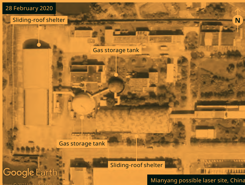
FIGURE 17-29 — LASER TEST SITE NEAR MIANYANG
