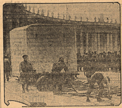
Here are eighty-six tons of marble being moved through St. Peter's square in Rome. It is the giant block which will serve as a base for the lofty monolith in the new Mussolini stadium which is under construction. Curved strips of cooped wood were used to transport the heavy block.
