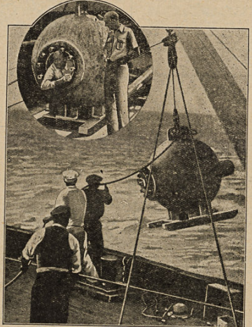
Steel ball containing Otis Barton, its inventor, and Dr. William Beebe, on its way down to nearly half a mile below the surface. Inset: Mr. Barton in bathysphere, Dr. Beebe beside it.
