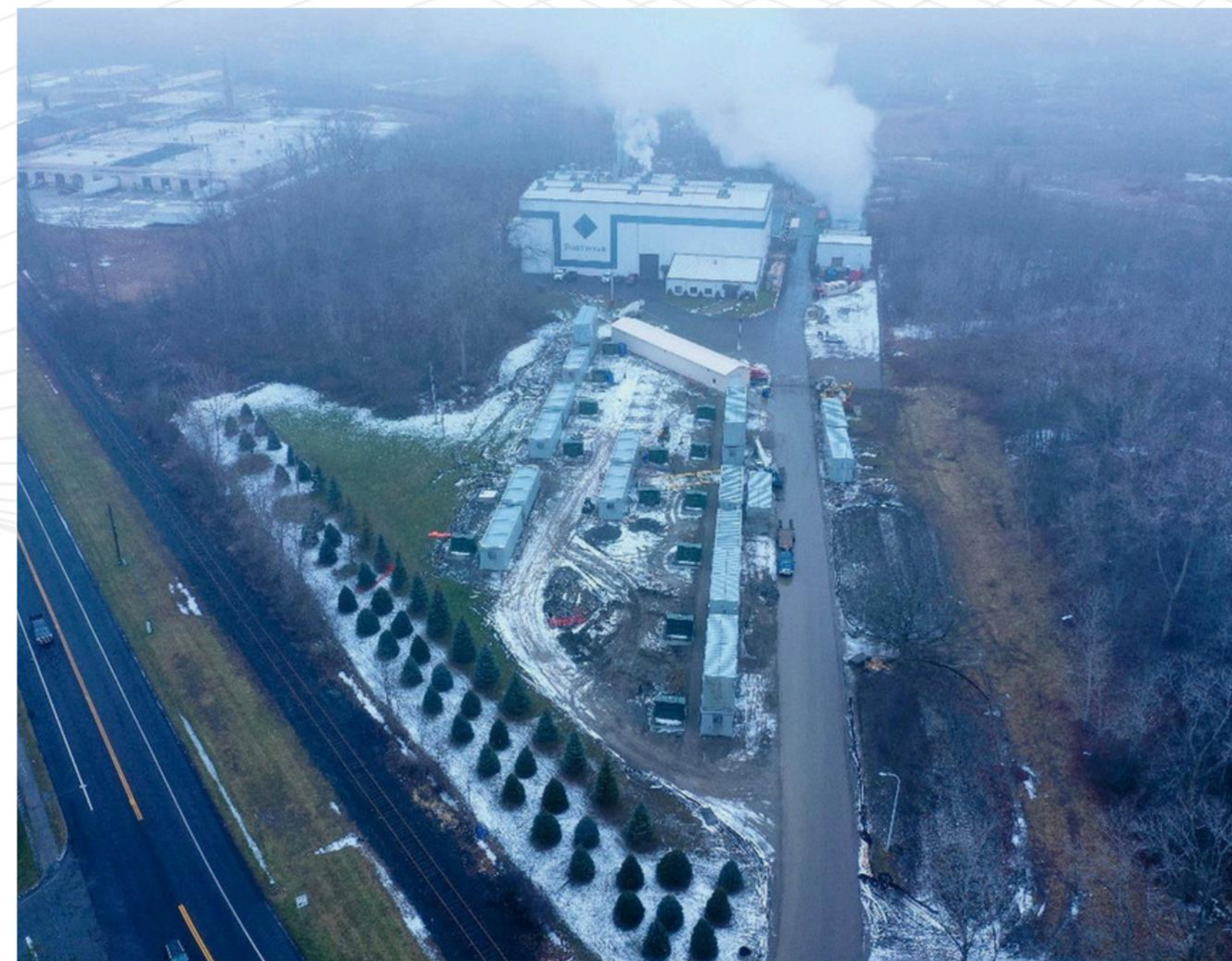
Arial View North Tonawanda PP
