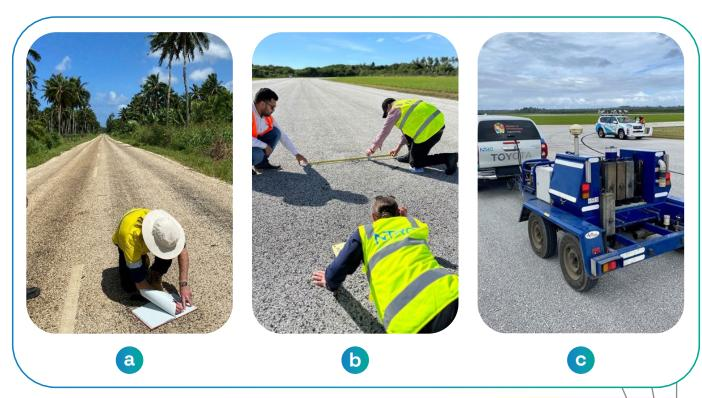
Figure 4: NTRO team undertaking (a) road inspections, (b) runway pavement inspections, and (c) FWD testing on runways for PCR assessment
