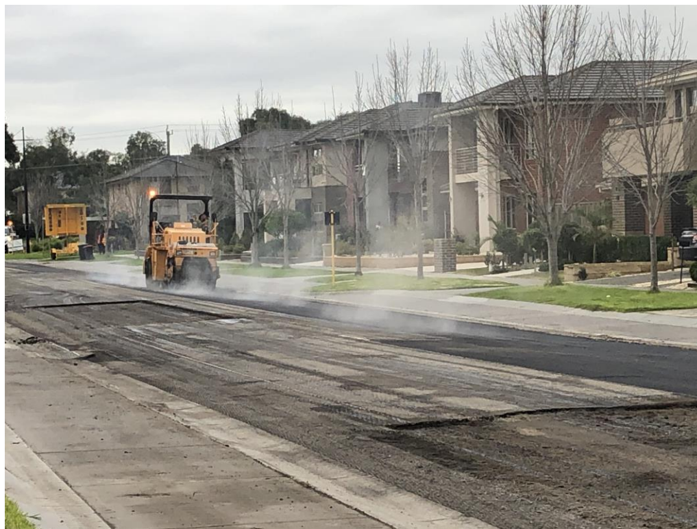
Figure 2 Church Road during construction – compaction
