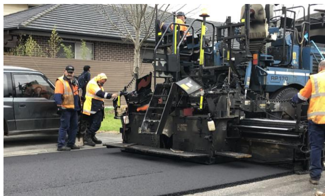
Figure 1 Church Road during construction – re-surfacing with 35mm depth 10 LTCRA
