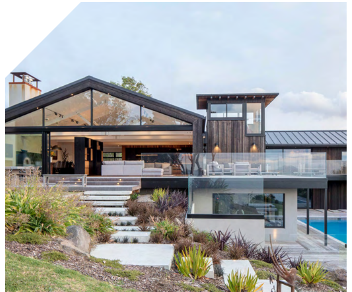
Whitford Home Extensive Renovation
