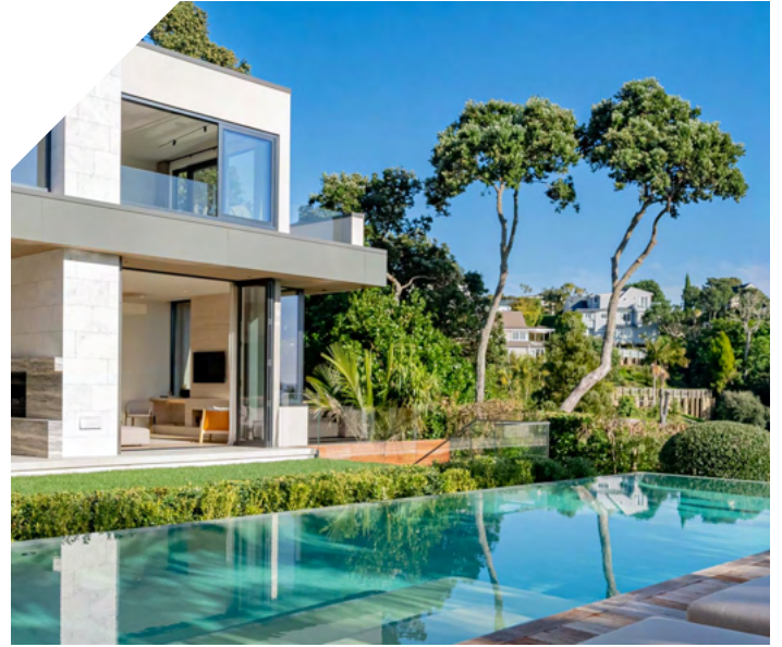
Remuera Home Extensive Renovation
