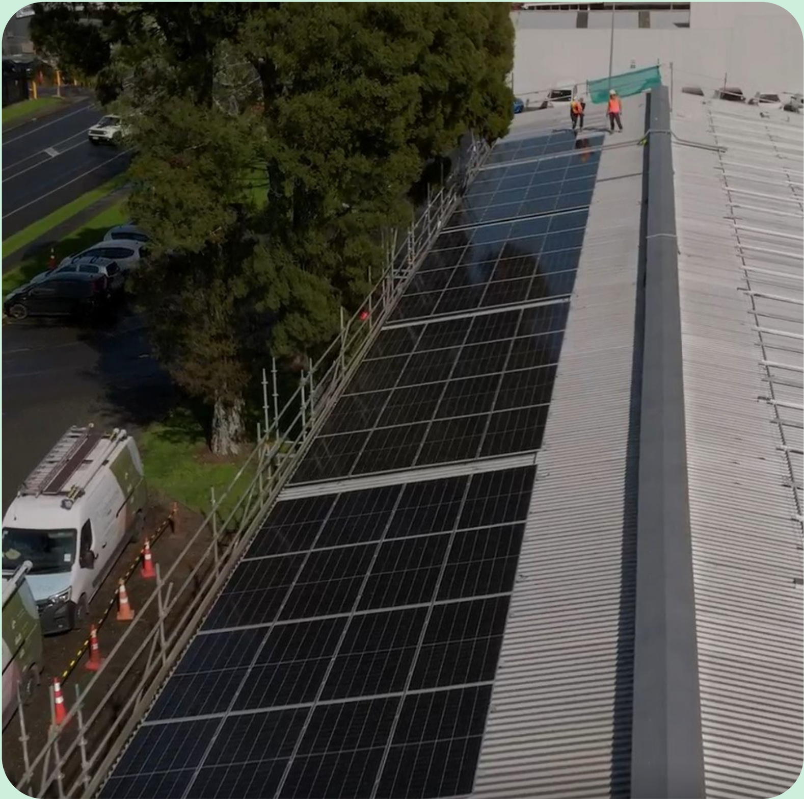
ABOVE Solar being installed at Counties Energy.
