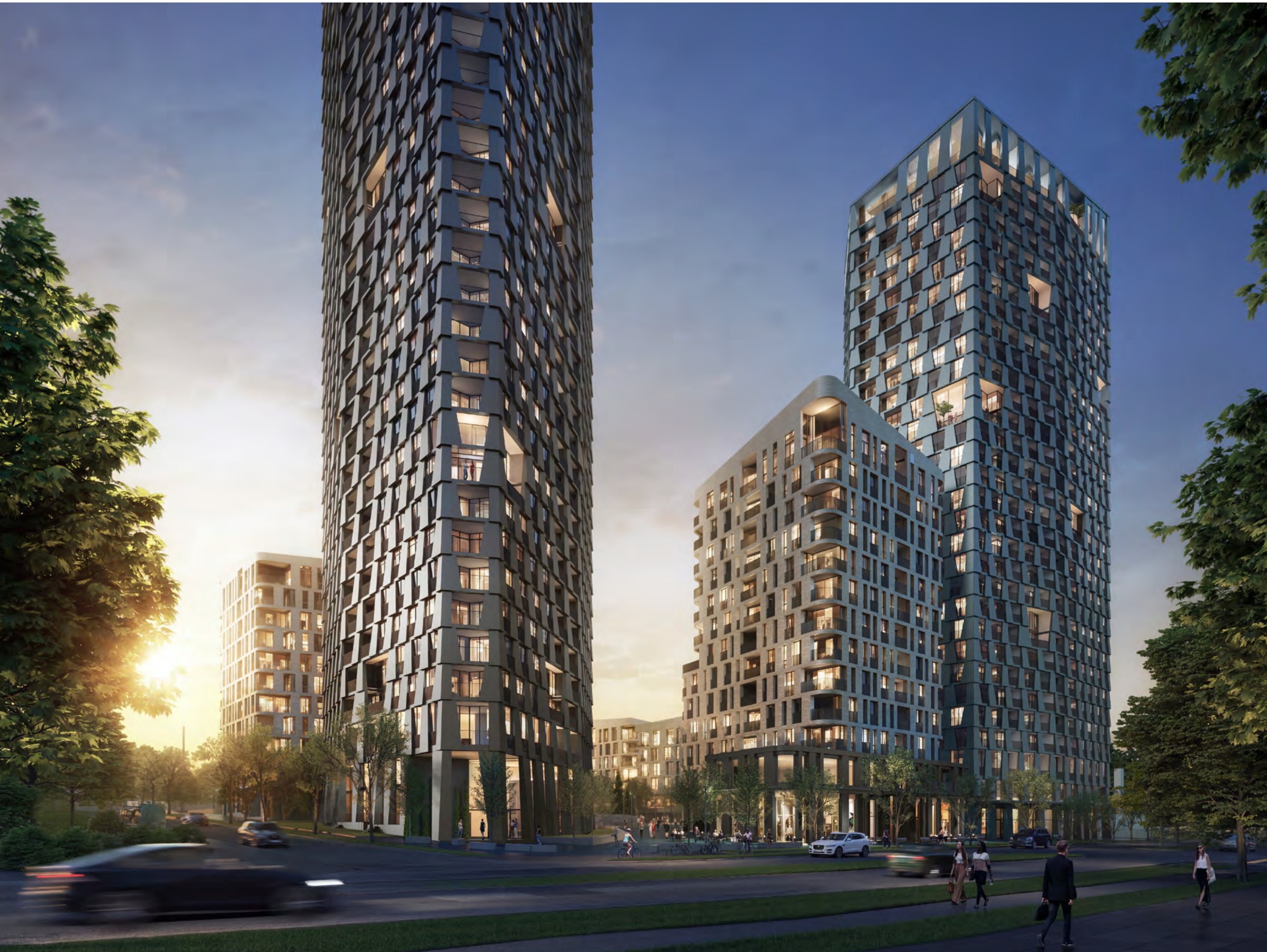
WHALLEY BOULEVARD VANCOUVER ALISON BROOKS ARCHITECTS LOCATION: LONDON, UK
