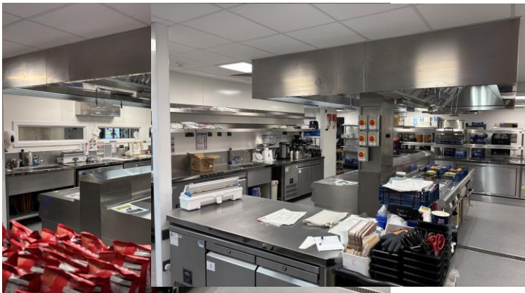
Commercial kitchen, preparation and production areas
