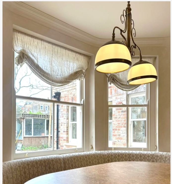
Box Sash Windows
