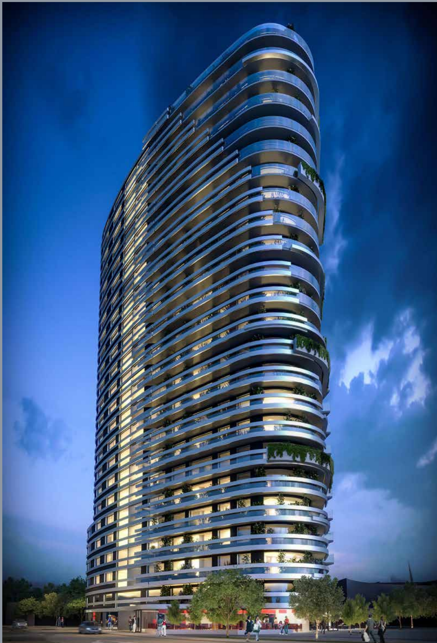
Image – The Pump House, 23-storey residential tower. Kitchens, furniture and doors installed in 161 apartments
