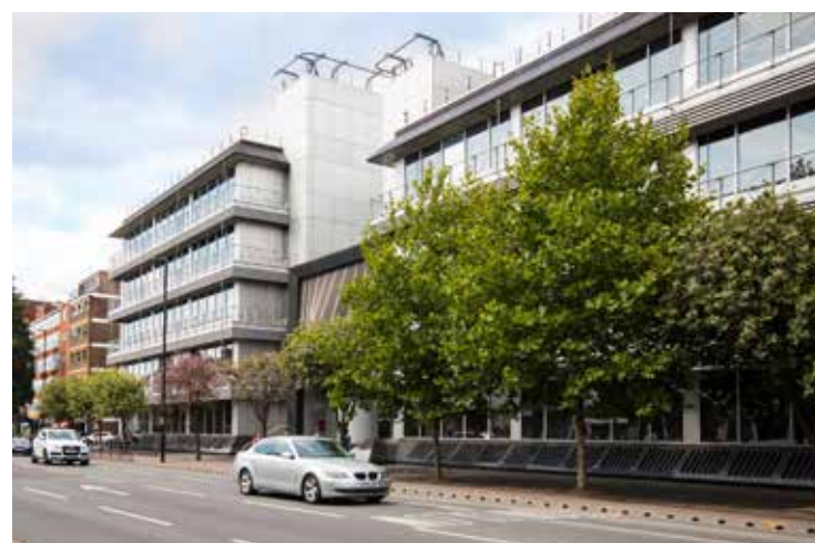
The conversion of an existing 6 storey office building under permitted development to 228 residential apartments. VPK supplied kitchens, wardrobes, vanity units and doors to each flat
