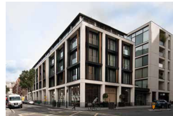
Bespoke joinery installed in 44 luxurious apartments and penthouses
