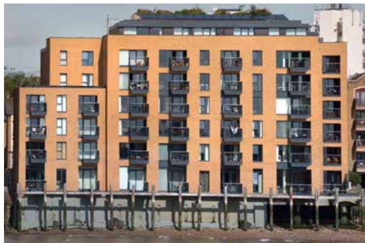
VPK supplied and installed a selection of joinery to 110 apartments
