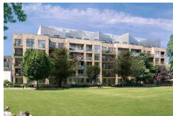
VPK supplied and installed wardrobes and vanity units to 60 luxury flats in Kilburn
