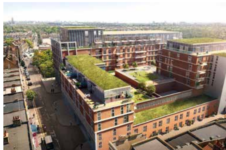
VPK supplied and installed kitchens, wardrobes, vanity units and doors to 178 apartments
