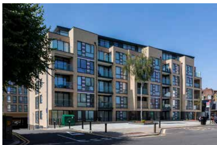
VPK supplied and installed 126 kitchens, 181 vanity units and 164 wardrobes
