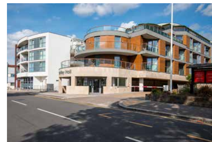
A selection of joinery was supplied and installed to 68 apartments which included kitchens, wardrobes and vanity units
