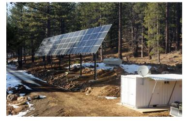
• **Solution**: A 97% renewable grid-tied microgrid was implemented, featuring 20kW of PV, 69kWh of BESS, and backup propane generation. The system provides peak demand
