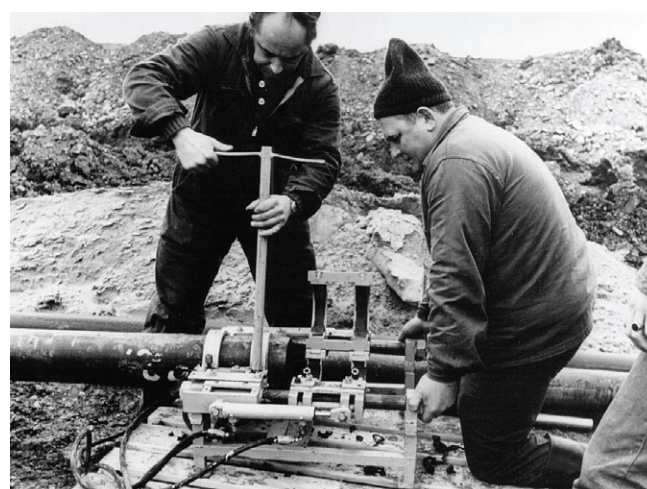
A Polybutene piping installation over 50 years ago
