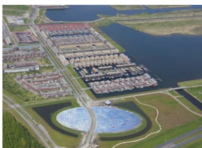
District Heating - Almere, NL
