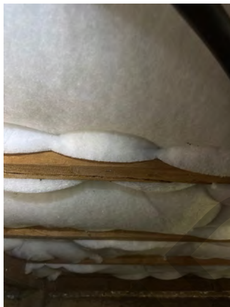
Some gaps in polythene membrane in places.
