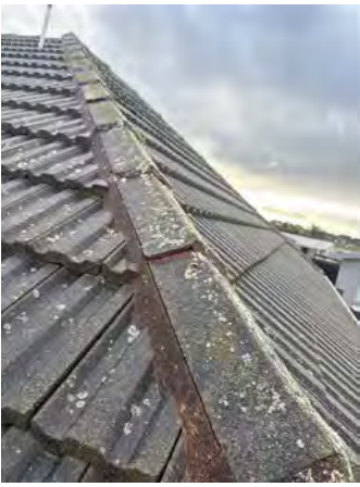
Example - typical cracking and separation to mortar on tile hips and ridge capping throughout.
