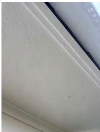
Close up example of notable weathering to some sections of soffit.
