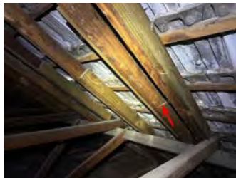
Example - rafters have been cut throughout and reinforced.
