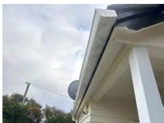
Close up example of notable weathering to some sections of soffit.
