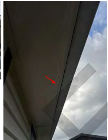
Splitting to scotias here.
