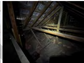
Vertical supports have been cut and reinforced.
