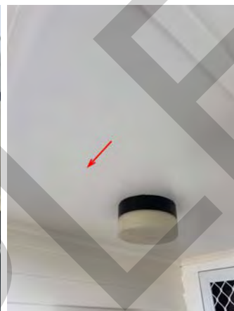
Crack in soffit.
