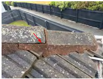
Example - typical cracking and separation to mortar on tile hips and ridge capping throughout.
