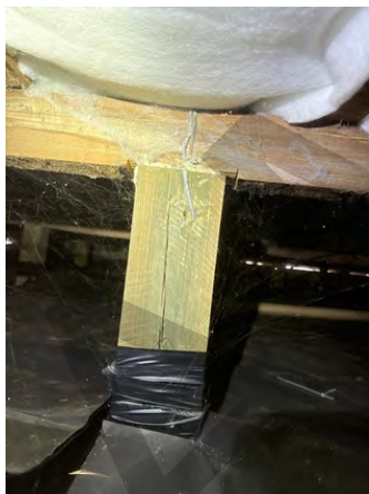
Monitor split pile.
