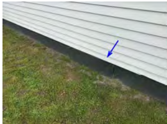
Sub floor access on the NE exterior wall.
