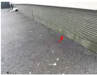
Example - fibre cement finishing below ground level.
