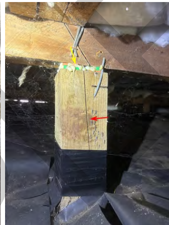
Split pile and example of precast packers.
