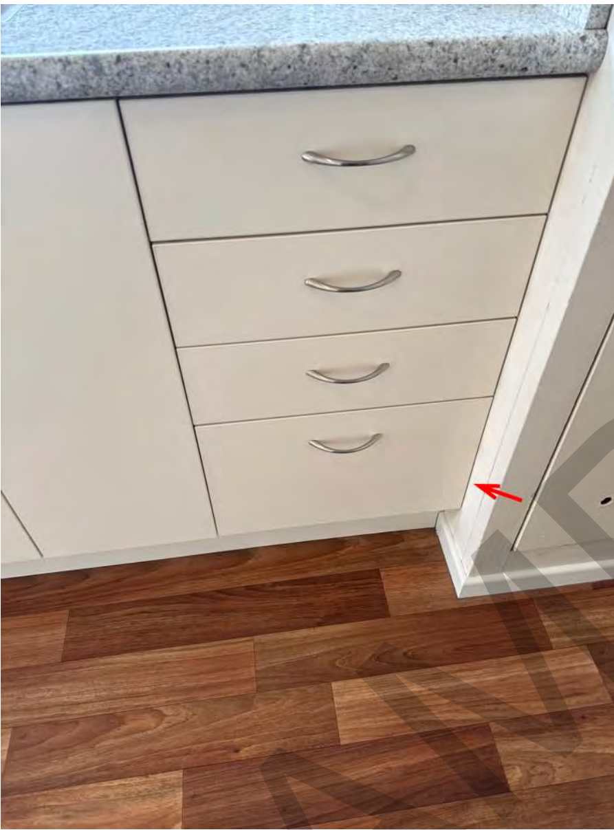
Bottom drawer catches slightly.
