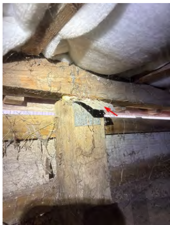
Re-attach nail plate.
