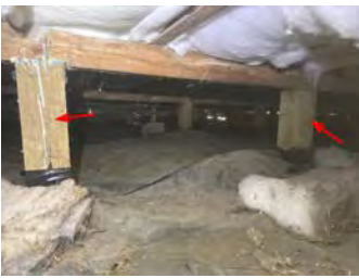
Split piles. One has been glued together.
