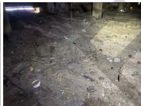
Some gaps in polythene membrane in places.
