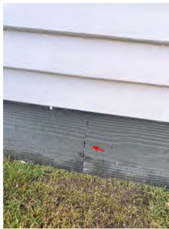
Cracked board.
