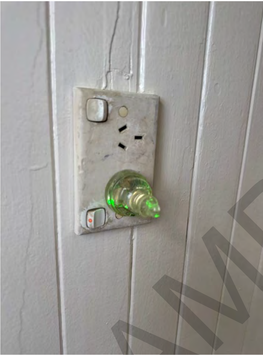
Example of test carried out.
