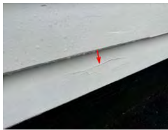
Example - some splitting to paint.
