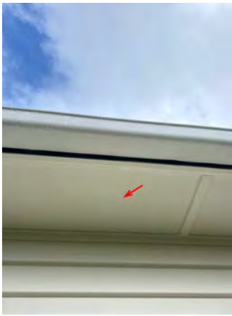
Cracked soffit.
