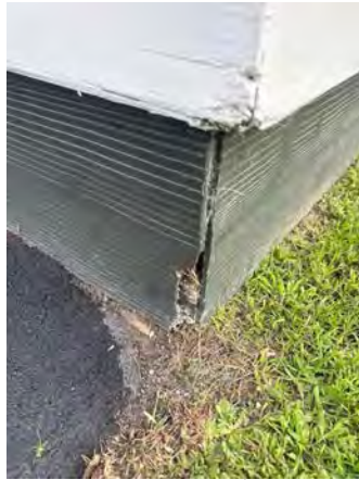
Cracked board.
