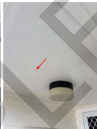
Crack in soffit.
