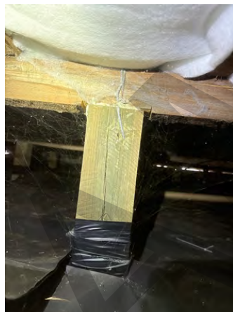
Monitor split pile.
