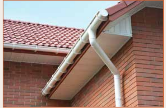
Install gutters at the edge of the roof
