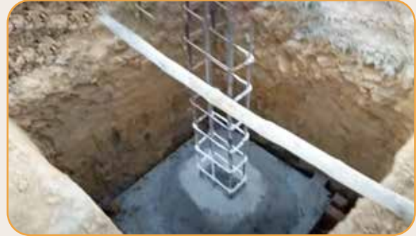
Concrete poured & shuttering
