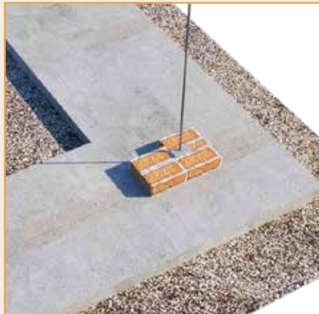
Single steel bar reinforcement at junctions
