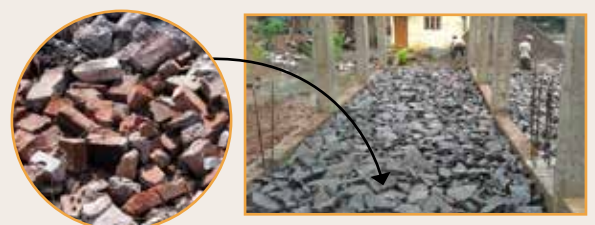
Debris Materials can be used for plinth filling
