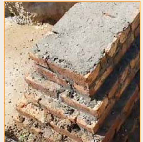
Stepped brick foundation
