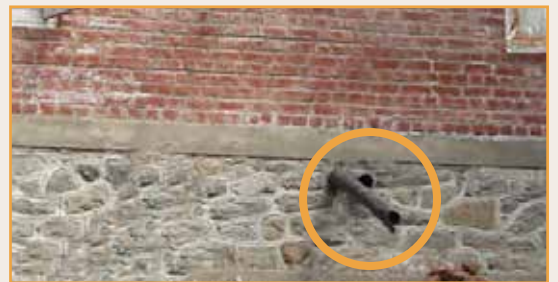
Provide plumbing outlets while laying the plinth
