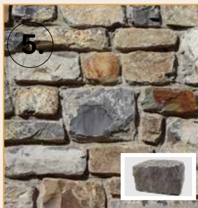
Masonry with local dressed stone & mortar
