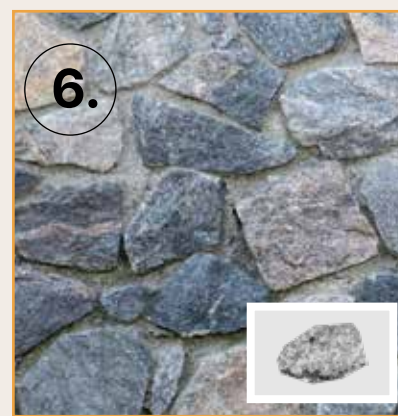
Random Rubble Masonry with local stones & mortar
