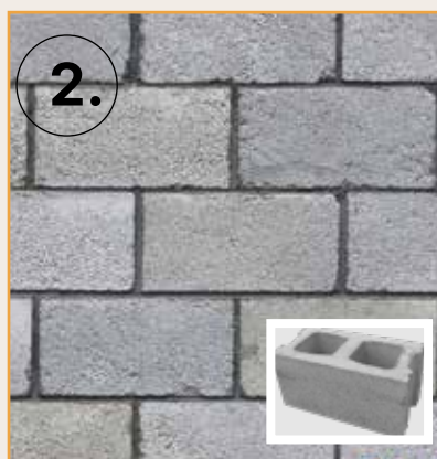
Masonry with concrete block and mortar
