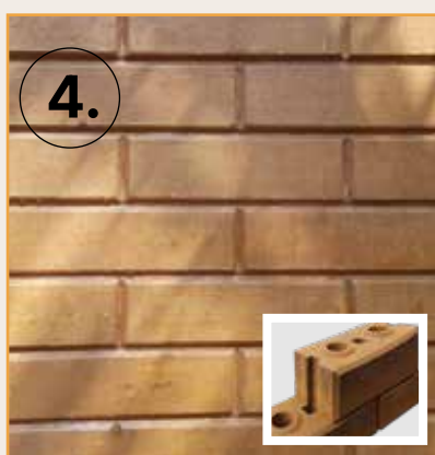
Walls with CSEB or 'Compressed Stabilized Earth Blocks' & mortar
