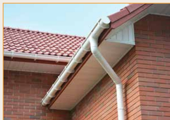
Sloping roof & its drainage
