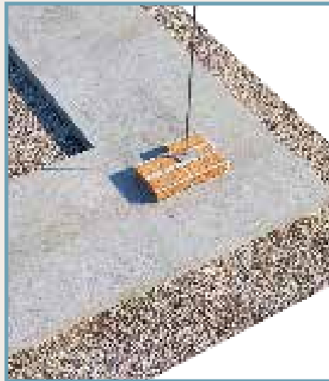
Single steel bar reinforcement at junctions
