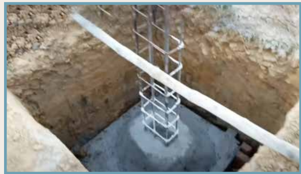
Concrete poured & shuttering
