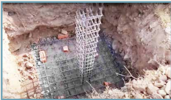
Steel cage positioned on PCC base using spacers
