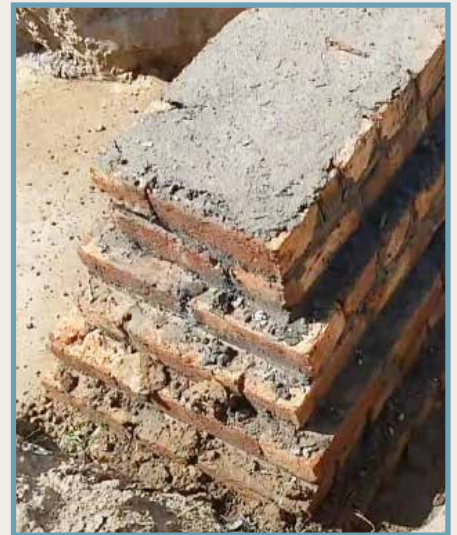
Stepped brick foundation
