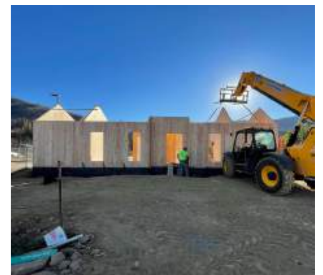
Wet-core prefabrication & on-site mass timber assembly Construction photos courtesy of atelierjones
