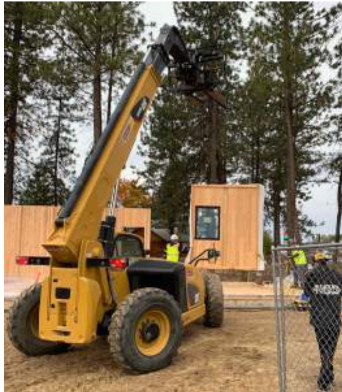
1 On-site installation of prefab walls
