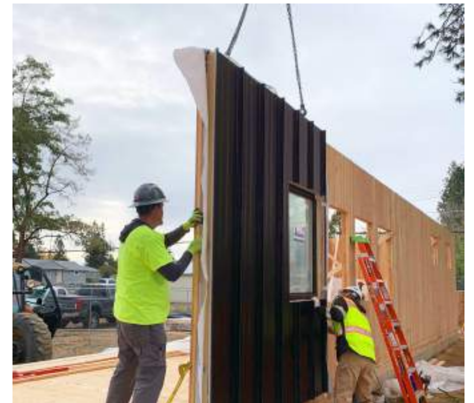
7 Prefab CLT wall assembly
