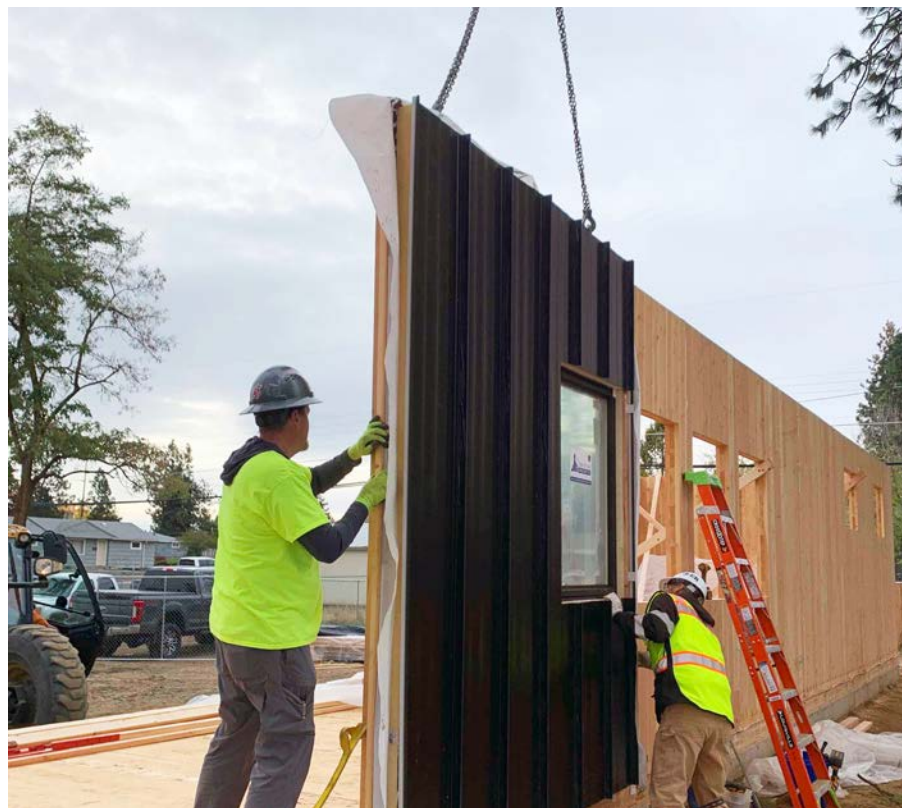
5 Prefab CLT wall assembly
