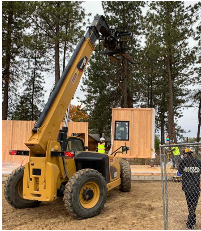
1 On-site installation of prefab walls
