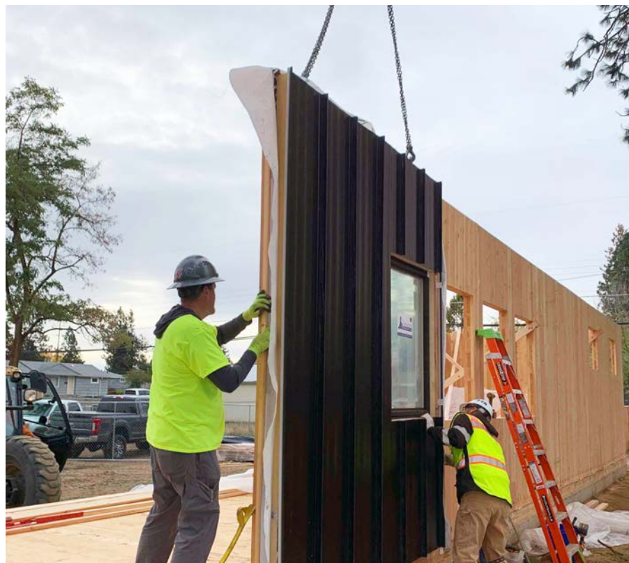
5 Prefab CLT wall assembly
