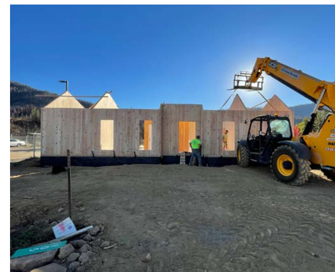
Wet-core prefab & on-site mass timber assembly Construction photos courtesy of atelierjones
