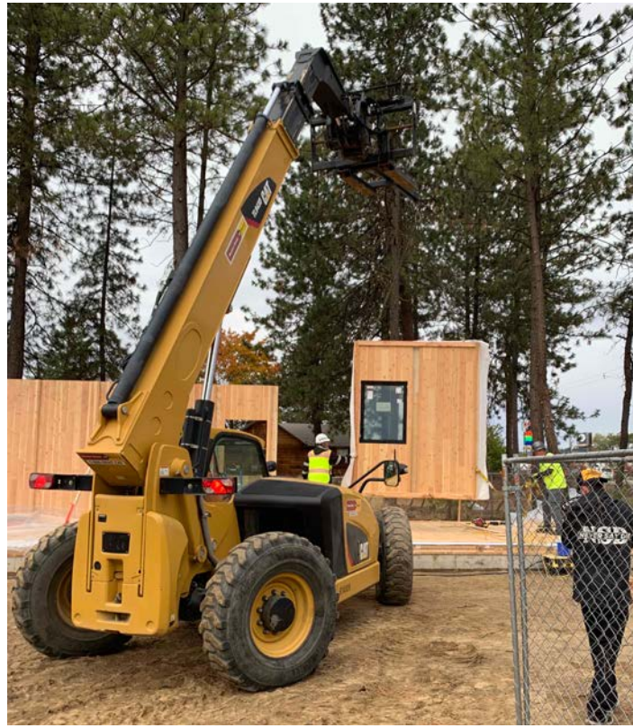
1 On-site installation of prefab walls
