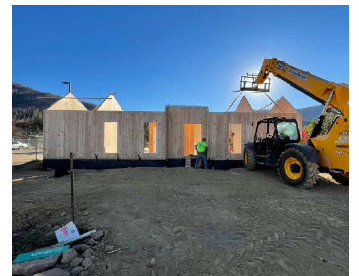
Wet-core prefab & on-site mass timber assembly Construction photos courtesy of atelierjones
