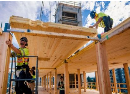
EMTC Facade, Point-supported CLT, and Concrete
