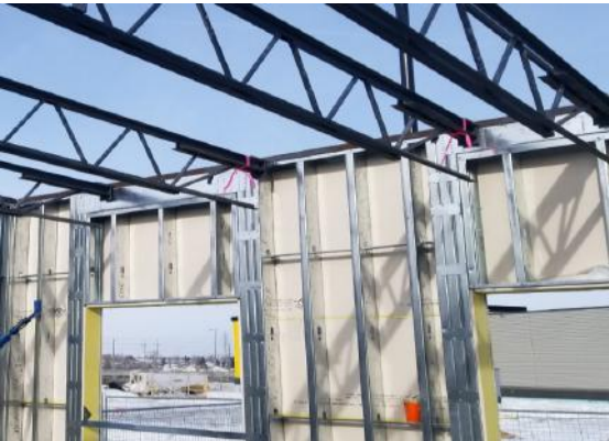
Steel stud, Steel Web Joists, and Concrete
