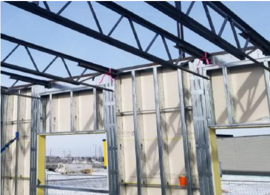
Steel stud, Steel Web Joists, and Concrete
