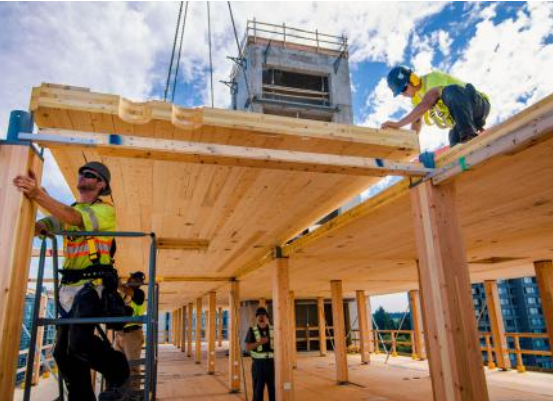
EMTC, Facade, Point-supported CLT, and Concrete
