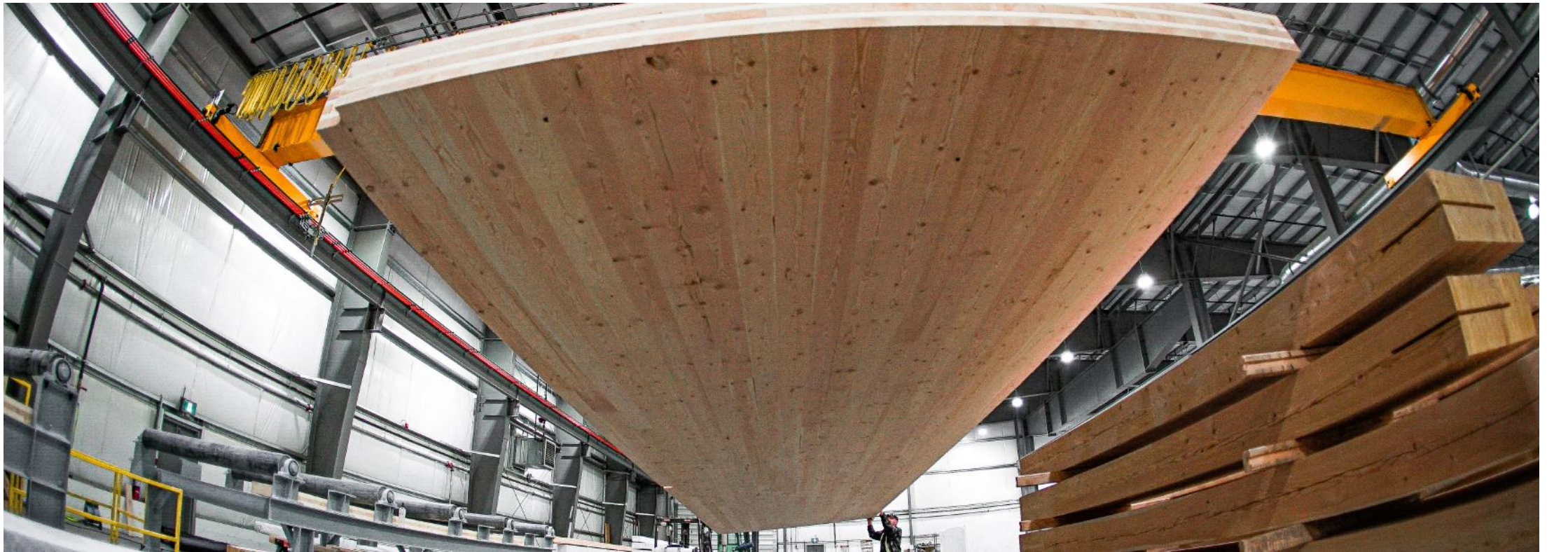
Photo of CLT CNC Fabrication. (Kalesnikoff)
