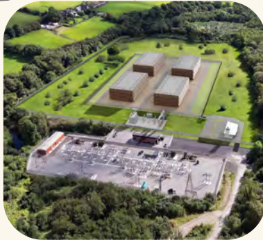
Last Energy Power Plant
