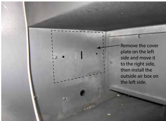
Figure 3.14 Remove Cover Plate (Left Side)
