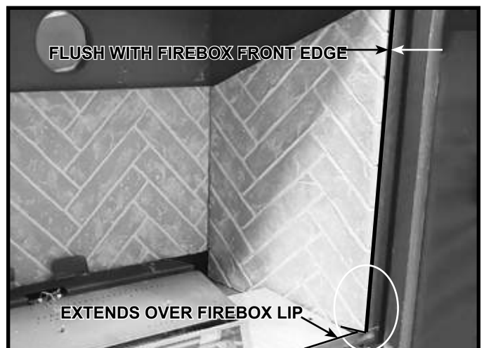
Figure 11.4 Side Refractory Panel Installed (Right Side Shown)
