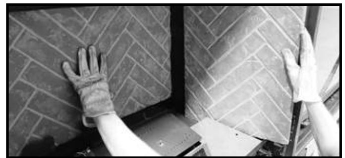
Figure 11.3 Install Side Refractory Panel (Right Side Shown)
