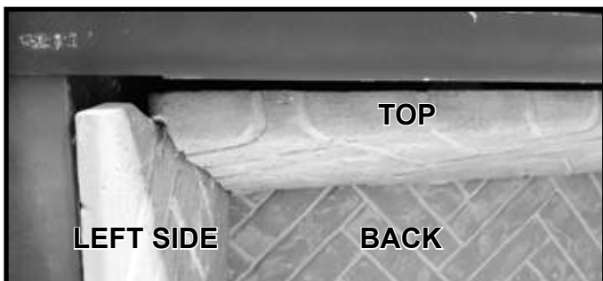
Figure 11.5 Install Top Refractory Panel - Left Side Shown
