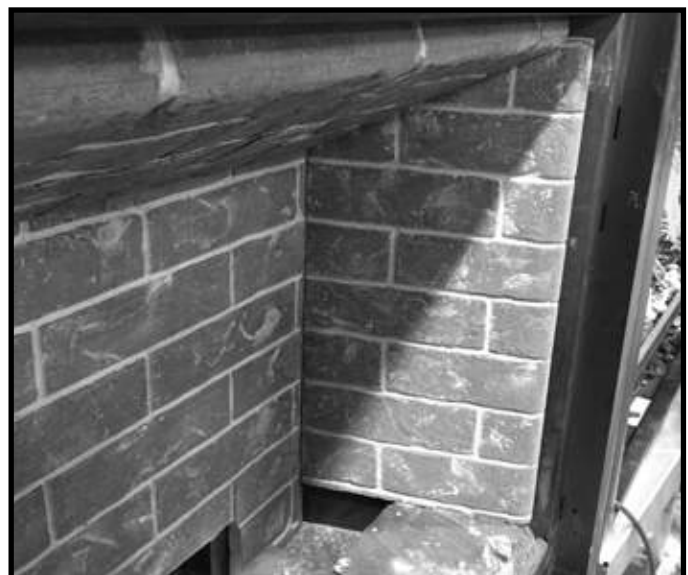
Figure 11.6 Right Refractory Panel Installed
