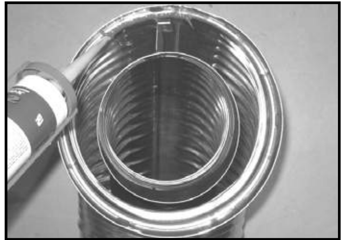
Figure 7.1 High Temperature Silicone Sealant
