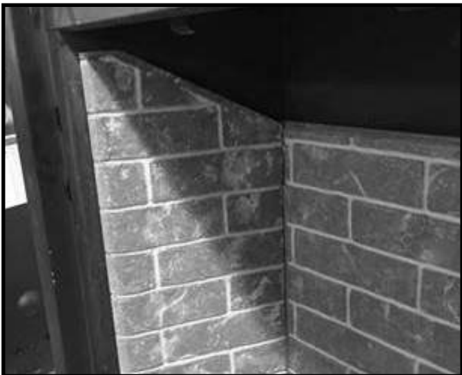
Figure 11.3 Install Left Refractory Panel
