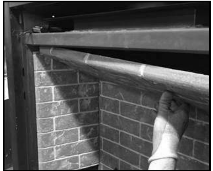
Figure 11.4 Install Top Refractory Panel
