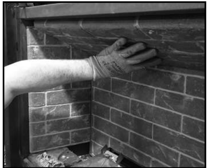
Figure 11.5 Install Right Refractory Panel
