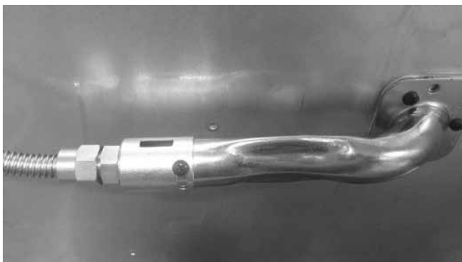
Fig 9.1 Air Shutter Natural Gas
