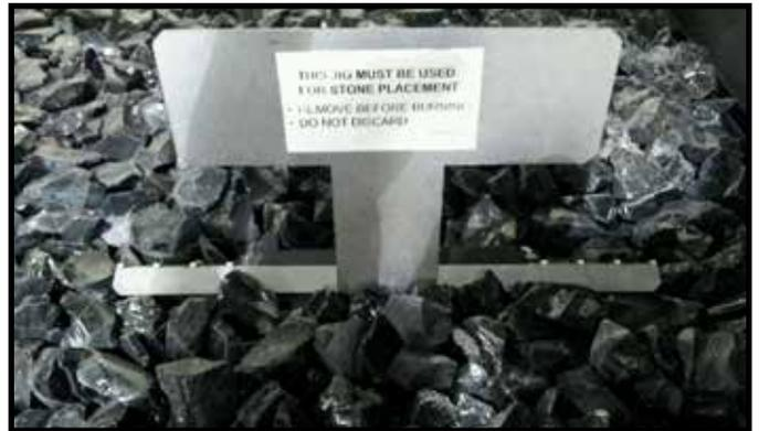
Figure 9.9 Rock Placement Jig
