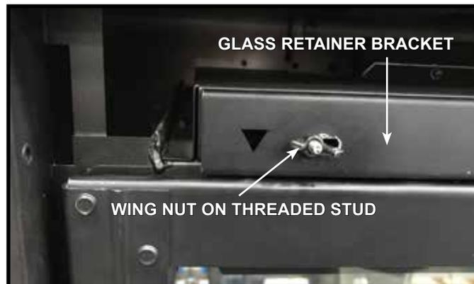
4.3 Glass Retainer Bracket & Wing Nut Detail
