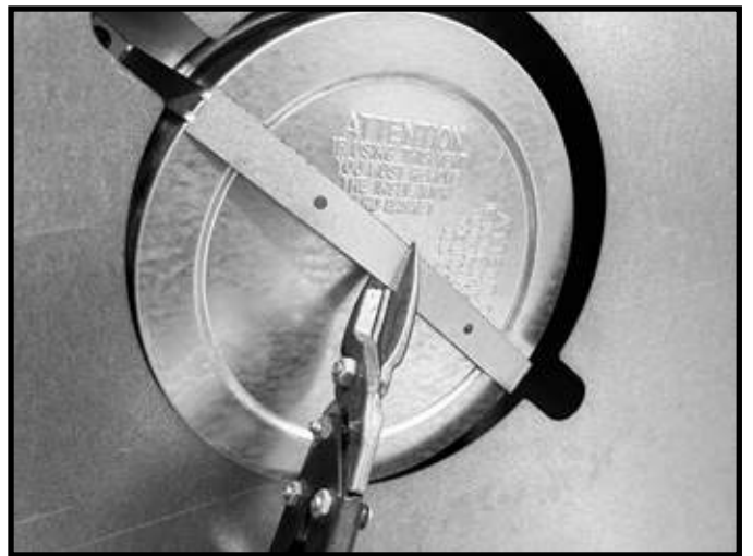
Figure 6.13 Cut the metal retaining band.
