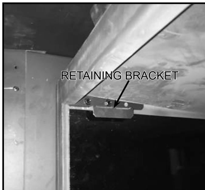
Figure 5 Retaining Bracket Installation - Side Panel
