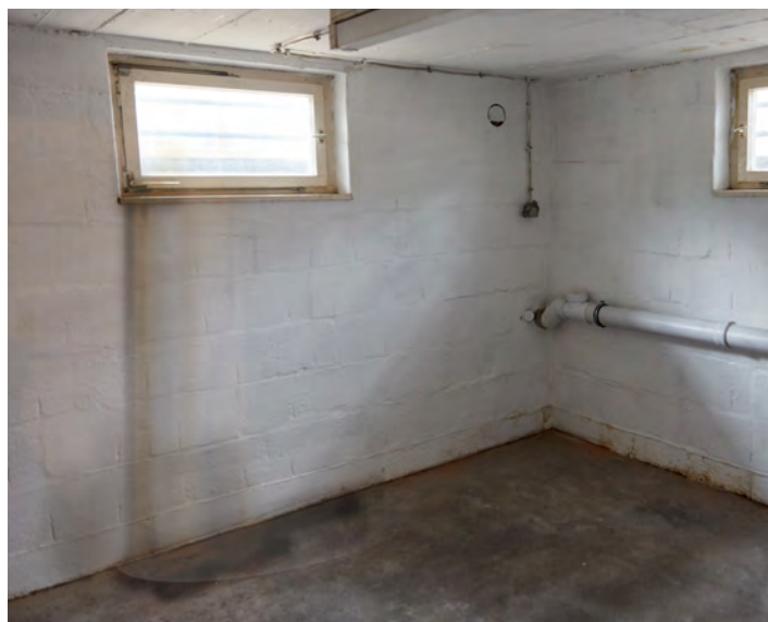
Unaddressed basement window seepage can lead to standing water, damp and humid air, odor, mold and mildew.
