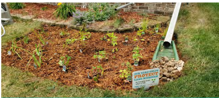
Disconnected downspout empties into a rain garden. Source: MMSD
